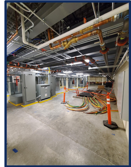
Completed CRAC Lineset
